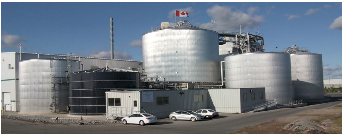
Toronto, Canada – Disco Road Organics Processing Facility, Anaerobic Digester https://www.biocycle.net/toronto-expands-anaerobic-digestion-of-source-separated-organics/
