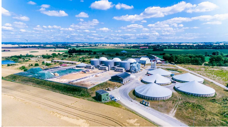
Jordberga Biogas Plant – Northeast of Trelleborg, Sweden
