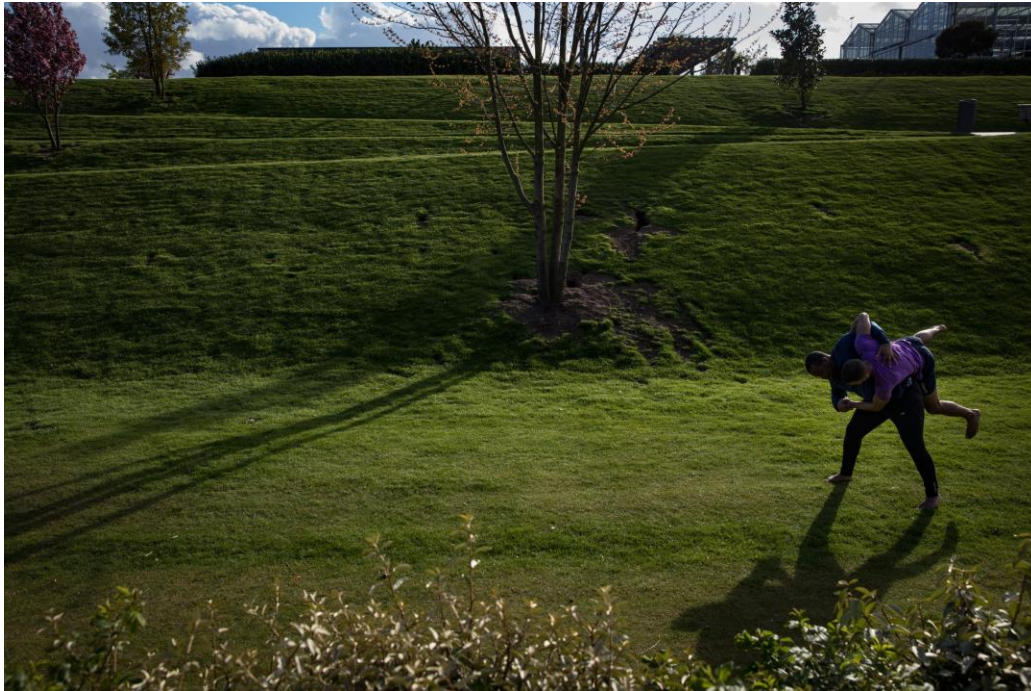
The Dakpark, a rooftop park incorporated into a dike in Rotterdam.
