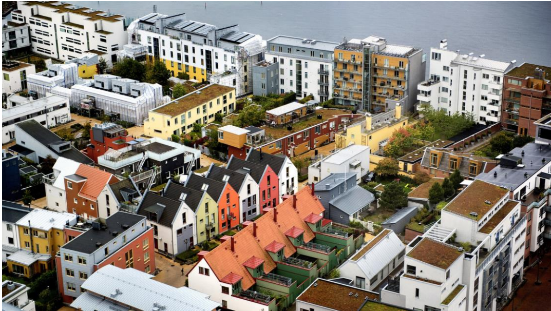
Västra Hamnen, once a decaying industrial area, has been transformed into a carbon-neutral neighbourhood – a prime example of sustainable city planning. Photo: Aline Lessner/ www.imagebank.sweden.se
