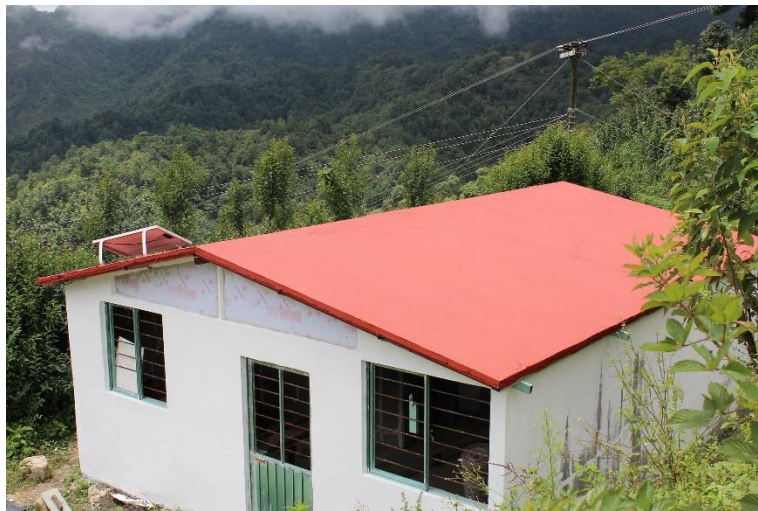
An EcoDom prototype house built using its plastic panels.
