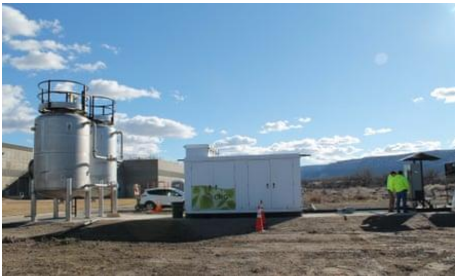
Vehicles wait to refuel at the Persigo Wastewater Treatment Plant in Colorado. Photograph: City of Grand Junction
