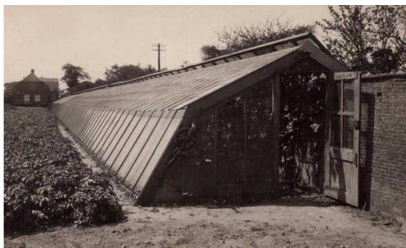
A Dutch greenhouse from the 1930s, built against a brick wall. Picture: Naaldwijk in oude ansichten .
