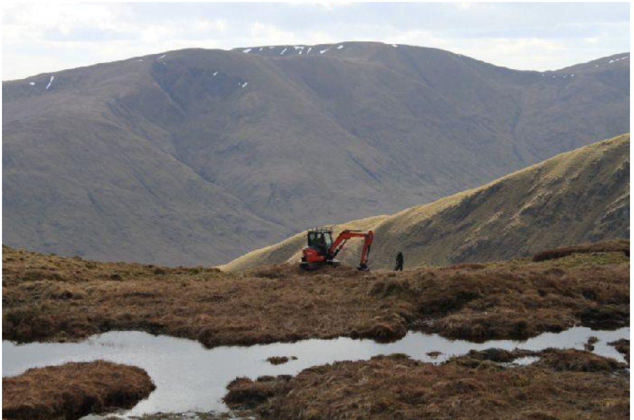
A bog pool, created by damming, at Beinn Dubh. Picture: Alan Bell
