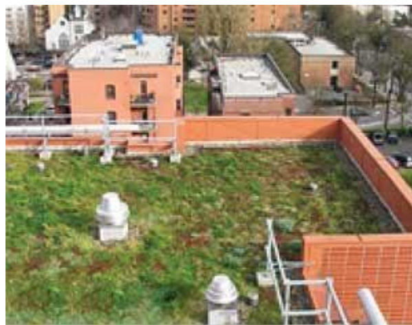
A green roof on an apartment building in Portland, Oregon. (Photo courtesy of Portland Bureau of Environmental Services)
