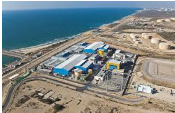
Sorek Desalination Plant. Credit: Photo courtesy of IDE Technologies
