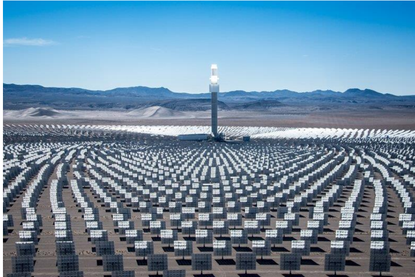
The 110-megawatt Crescent Dunes Solar Energy Facility in Nevada is the first utility-scale concentrating solar plant that can provide electricity whenever it's needed most, even after dark. Credit: SolarReserve
