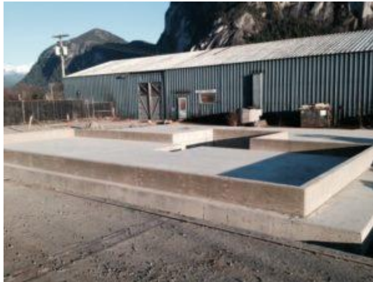
Carbon Engineering's carbon capture plant in Squamish. Carbon Engineering
