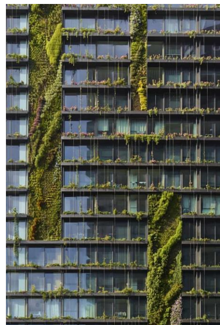
The side of One Central Park Sydney, showing the 1,120 sqm of vertical gardens. Photograph: Simon Wood/PR
