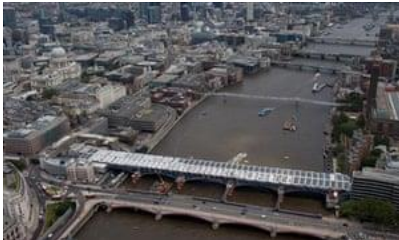
Blackfriars station solar panels installation underway in 2012. Photograph: Network Rail
