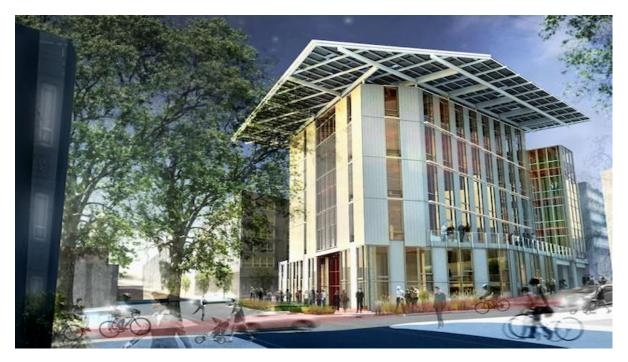
The 50,000-square-foot building will generate all of its energy using <u>solar panels</u>, and all of its water will be provided by harvested rainwater. There will be indoor composting toilets, a system of geothermal wells for heating, and the building's wood-framed structure is made out of Forest Stewardship Council certified wood.
