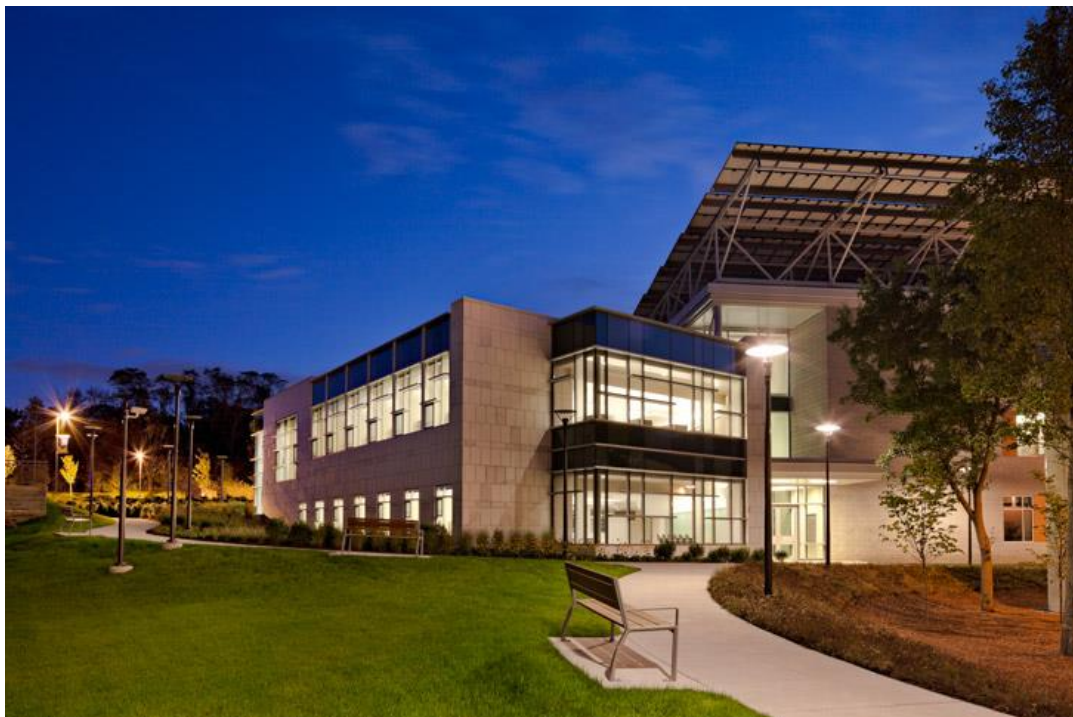
Efficient geothermal heat pumps, energy recovery units, grey water systems, high performance lighting, chilled beam technology, and a radiant heating/cooling system were all strategies that the team implemented to achieve a highly energy efficient building.
