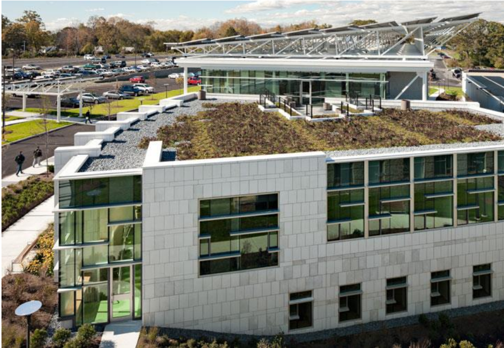
A green-roof system was also designed into exposed portions of the roof.
