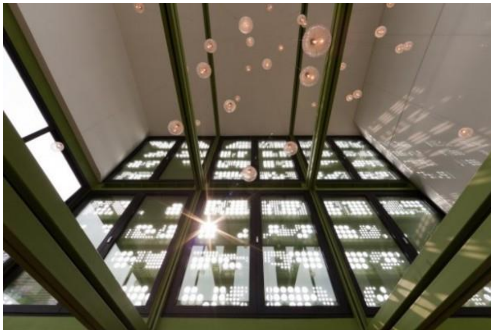
The doors of the containers have been perforated to provide a sun-filtering effect. Image by Bartosz Kolonko via Playze.
