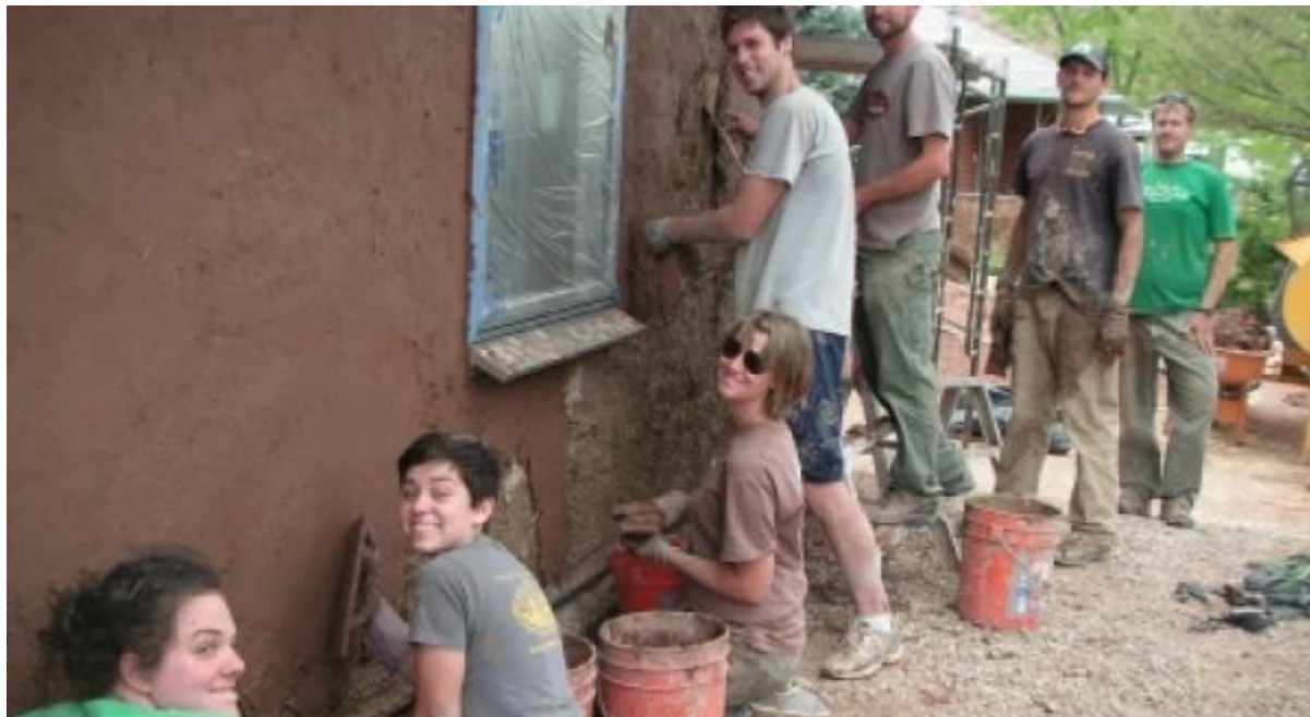
image via Community Rebuilds
