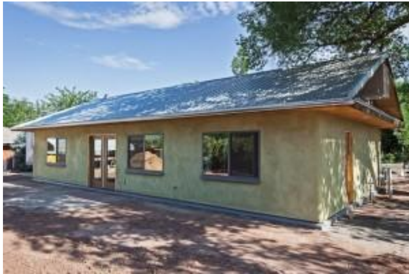
image via Community Rebuilds
